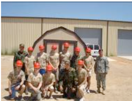
Finished Shed with Builders
